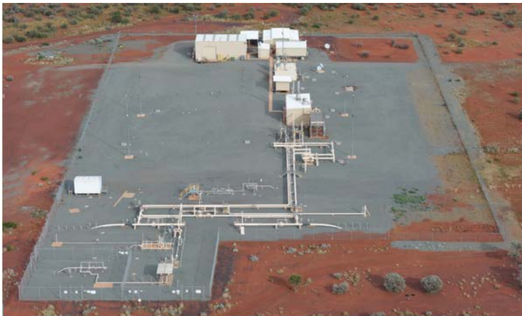
Photo. Wiluna Compressor Station
