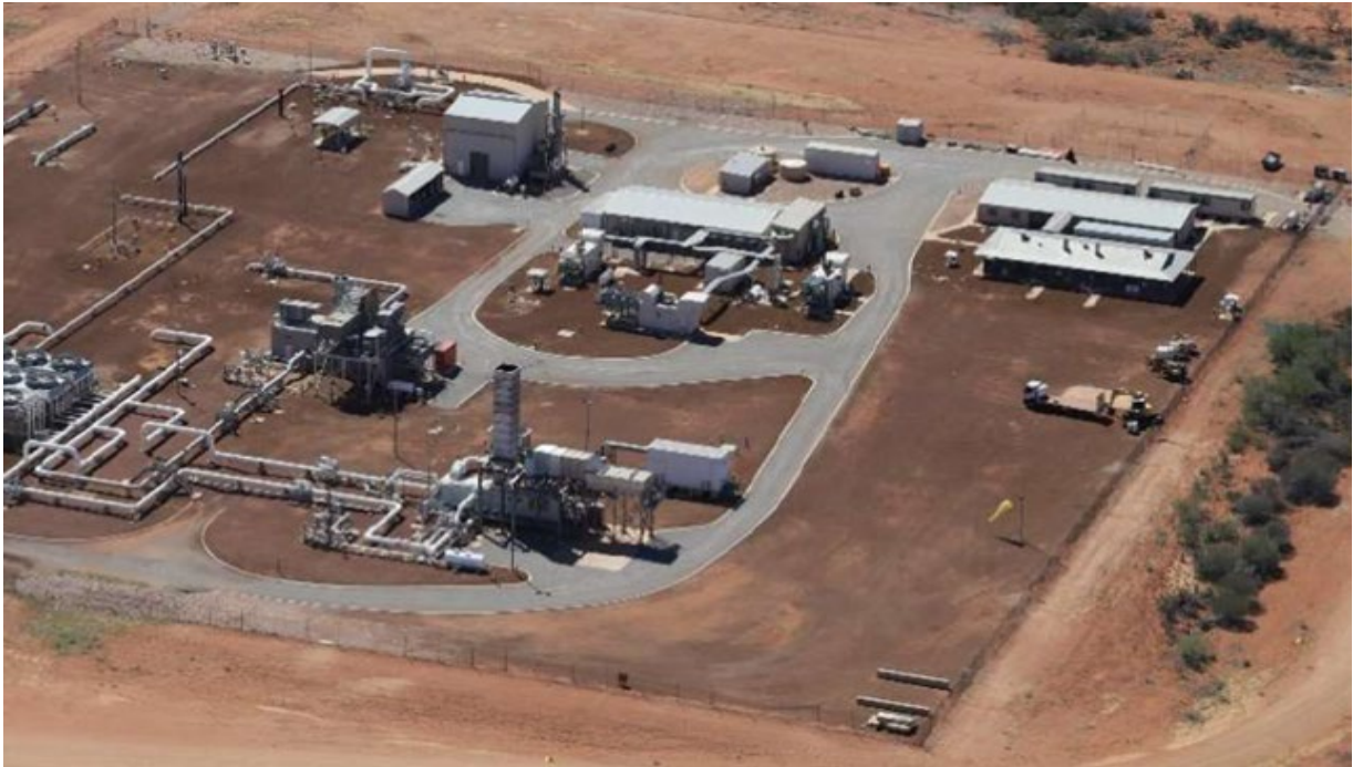
Figure 9.5: Operational site with accommodation near live assets and noisy operations.
