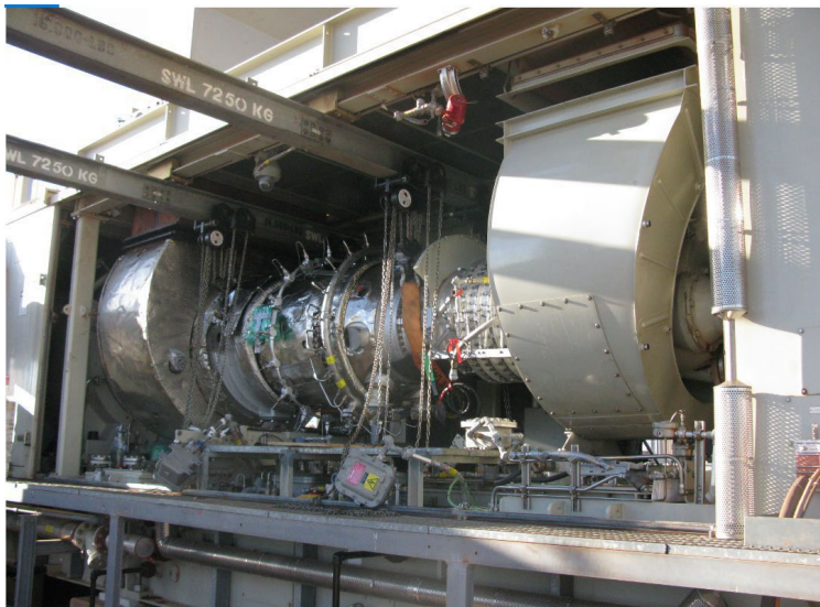
Figure 1.2: Gas turbine overhaul
