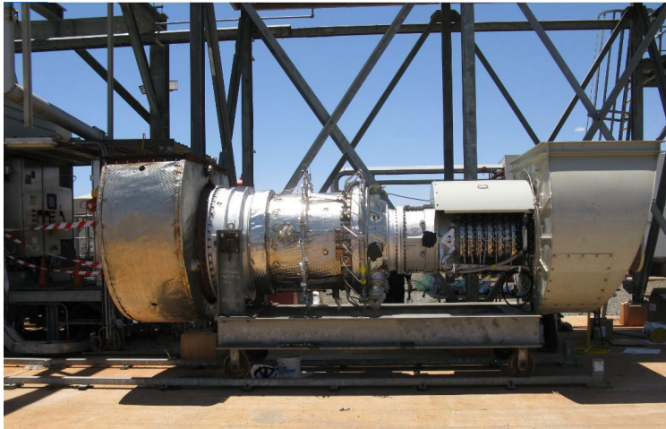
Figure 1.1: Gas turbine removal
