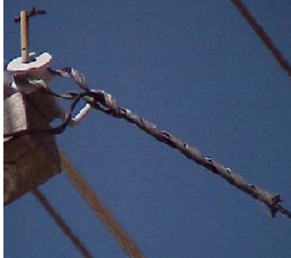
Figure 5: Example of a preformed steel termination (helical). The ends tend to perforate the insulation and become live and if the steel termination slips over the insulator, there is potential for the roof to become live and become a hazard.
