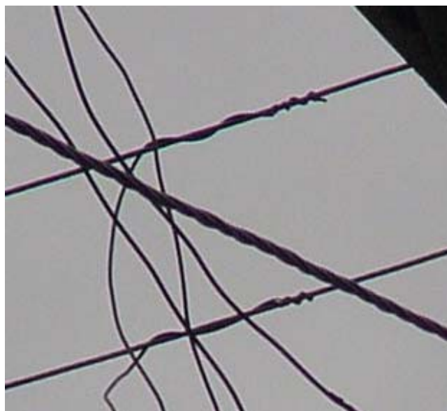
Figure 5: Example of a preformed steel termination (helical). The ends tend to perforate the insulation and become live and if the steel termination slips over the insulator, there is potential for the roof to become live and become a hazard.
