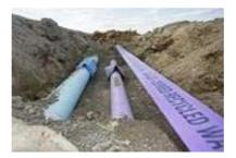
Drinking water pipe work will be marked 'drinking water' and coloured blue, with no obvious markings on the meter.
